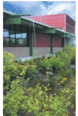
Figure 9 These disconnected roof leaders drop water into a bioretention/treatment area. Source: NRDC
