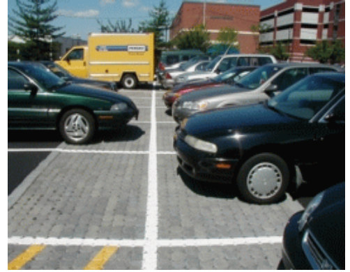
Figure 7 Permeable pavers can be installed in any low traffic flow area without reducing parking spots. Source: NRDC
